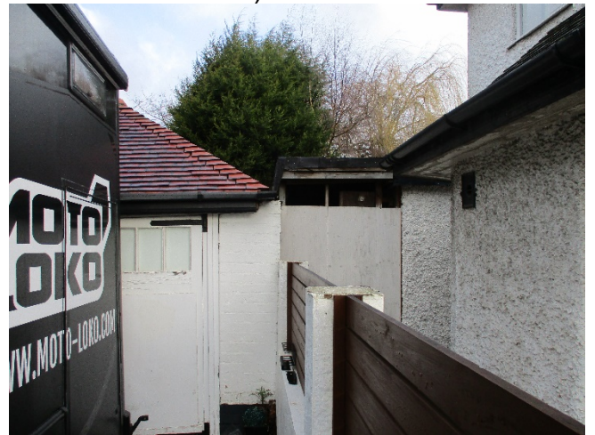
Site outbuilding and no. 114's store.
